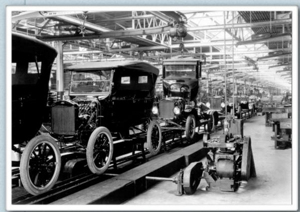
The car changed America FUFFEUEF. FORD'S ASSEMBLY LINE Henry Ford employs his assembly Line in Ford car plants nationwide THE ASSEMBLY LINE STANDARDIZED CAR PRODUCTION, MAKING IT FASTER AND CHEAPER TO PRODUCE CARS THIS TECHNOLOGY SPREAD TO OTHER INDUSTRIES, MAKING ALL GOODS CHEAPER AND MORE ABUNDANT
