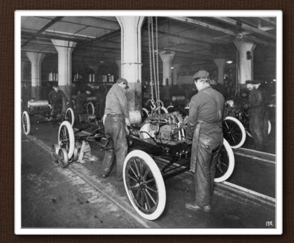
By OCTOBER 31, 1925, Ford plants produced 9,109 NEW MODEL-TS. That translates to ONE FOR EVERY 10 SECONDS OF THE WORKING DAY. With this kind of efficiency, Ford was able to lower the price from \$850 in 1908 to \$300 by 1926.
